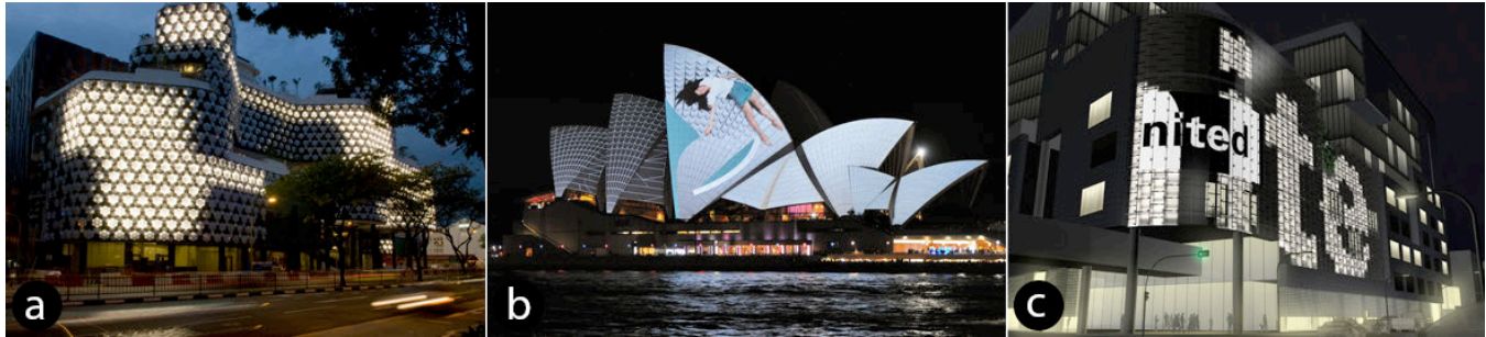
Figure 1: Examples of different media façade types in different locations: (a) Low-resolution light emitting façade type, (b) front-projection high-resolution type and (c) high-resolution screen embedded in a low-resolution light emitting façade. Image credits: (a) and (b): © realities:united, (c): © Jerry Dohnal.
